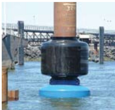
Pier pile fender
