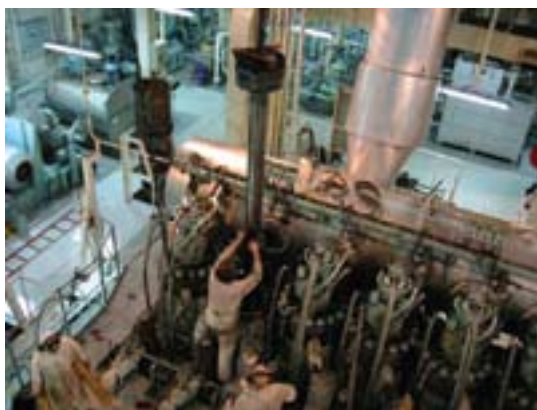
Overhauling piston no. 2.
