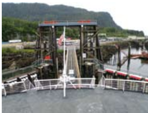
Link span with loading ramp
